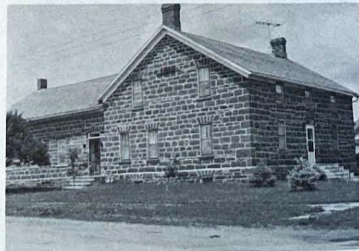
Typical Amanas sandstone block house built in 1862 and used as a communal residence.
