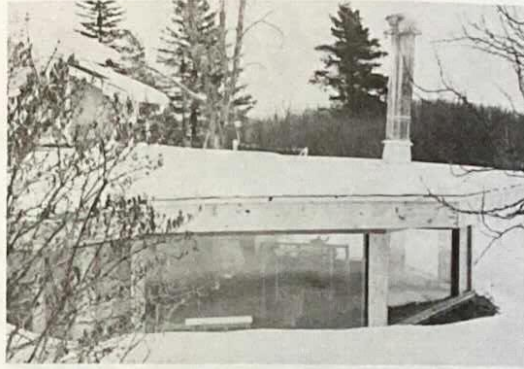
Thermopane windows allow lots of light and solar heat in Cathryn Miller's studio.
