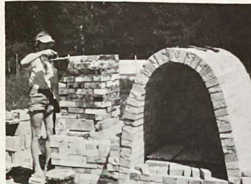
Working on the chimney.
